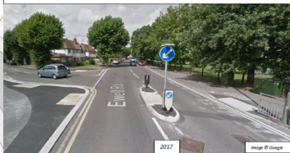
Ewell Rd/Rushett Rd Kerb build out and pedestrian refuge island
