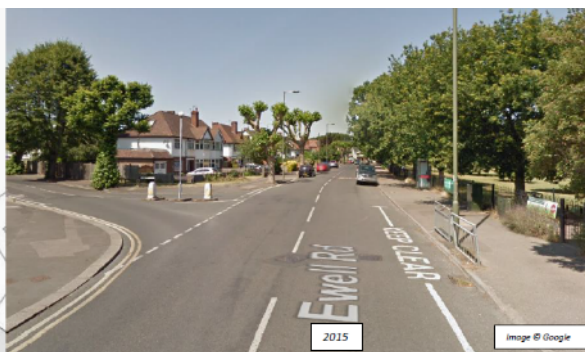
Ewell Rd/Rushett Rd Kerb build out and pedestrian refuge island
